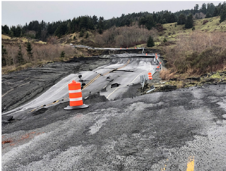
(left; Oregon) The Hooskanaden Landslide, triggered by heavy rainfall, caused substantial road damage. (right; Maunabo, Puerto Rico) Punta Tuna Wetlands Nature Reserve, which helps buffer the coastline from extreme events, was severely damaged during Hurricane Maria in 2017. Photo credits: (left) Oregon Department of Transportation [CC BY 2.0]; (right) Kenneth Wilsey, FEMA.
